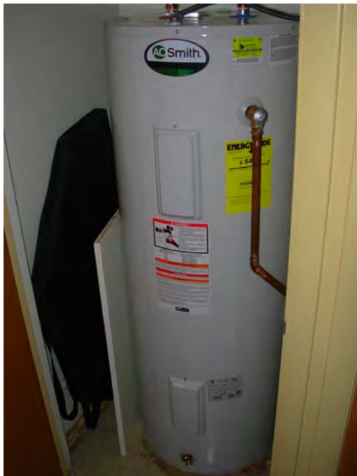
11. Domestic hot water tank serving community building Buckingham Terrace • Capital Needs Assessment • © On-Site Insight
