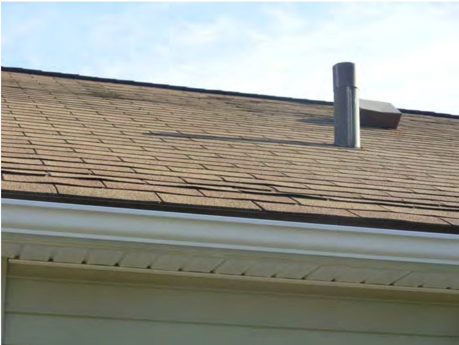
7. Spot lifting and curling of roofing shingles
