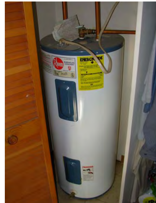
16. Electric DHW tanks serving all unit hot water needs
