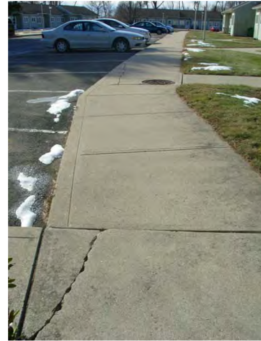
2. Concrete walkway cracking at spot locations
