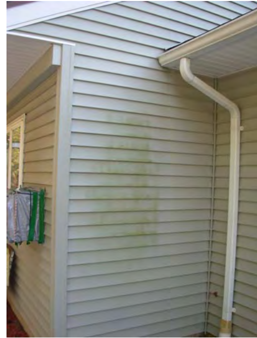
6. Organic material growth on some vinyl sided elevations
