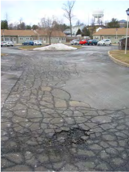
1. Asphalt paving, poor conditions observed
